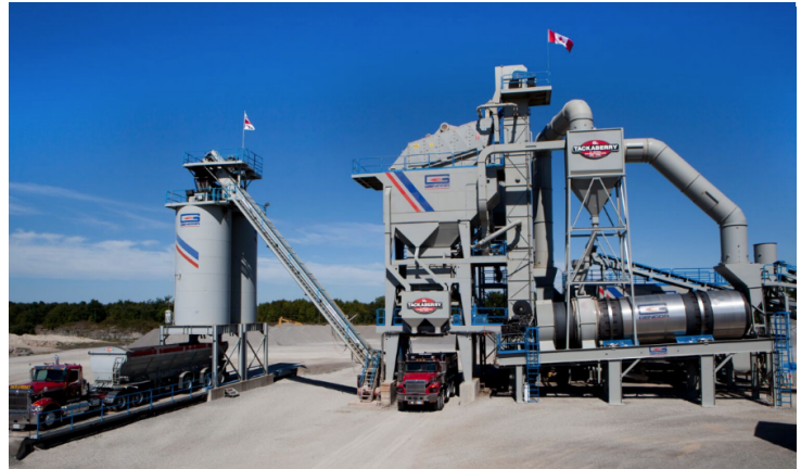
Figure 8: Gencor asphalt mixing plant
